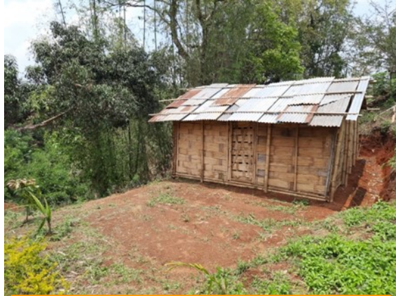
The Anganwadi (kindergarden school) constructed collaboratively this year.
